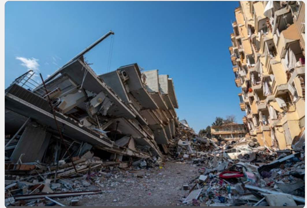
Wreckage of collapsed buildings after the 2023 Turkey-Syria earthquake
